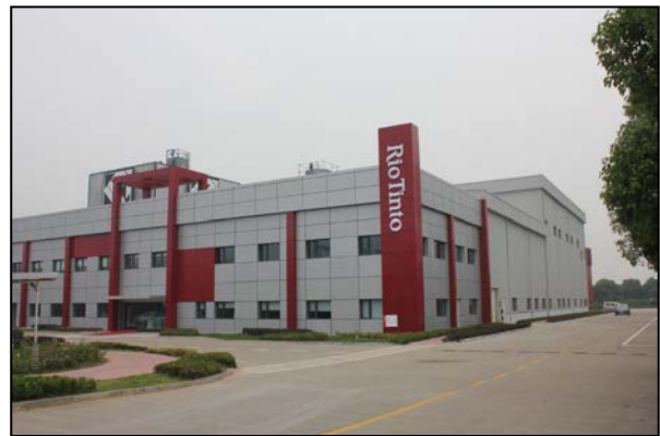
Rio Tinto QMP Metal Powders (Suzhou) plant
